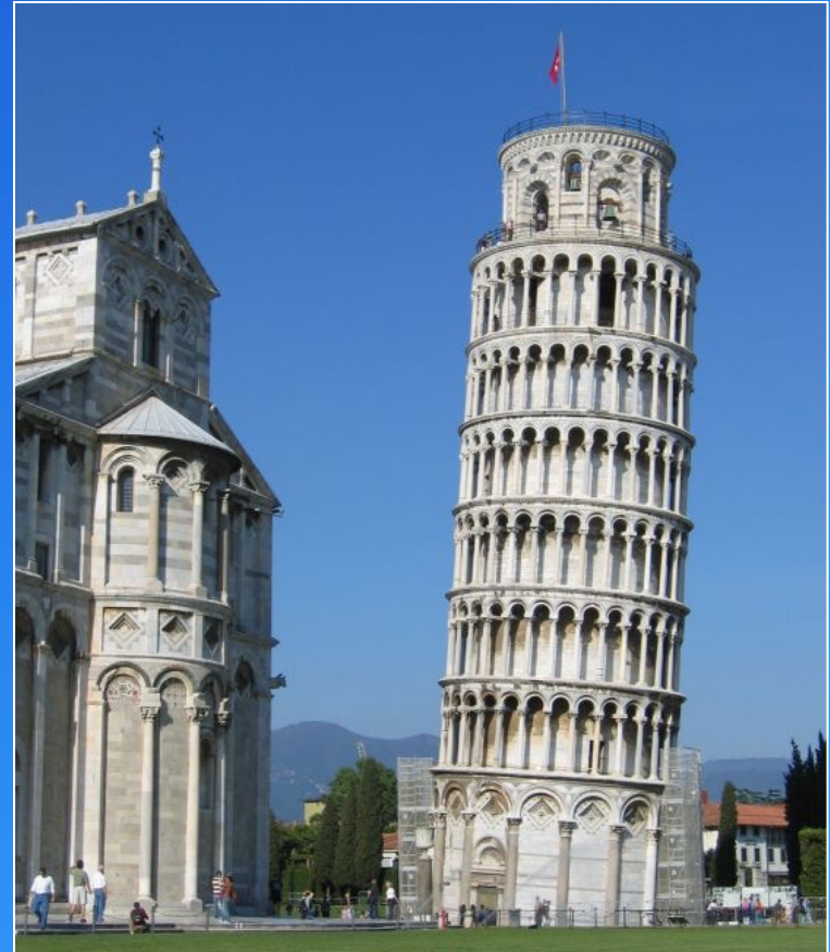
Tower of Pisa, Italy – inadequate foundation set in unstable soil. Wikipedia, 2010.
